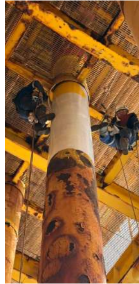
Humidur® FP applied with minimal surface preparation using power tools via abseiling activities on East Belulut Platform in May 2025
