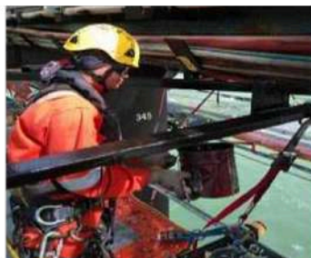
Humidur® FP products used for coating and repair of >100,000m 2 jetty structure and pipes using minimal surface preparation (dry ice blasting) during SPR2 Project at U 7200 in Brunei Darussalam from November 2017 - 2019
