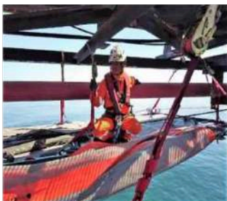
Humidur® FP products used for coating and repair of >100,000m 2 jetty structure and pipes using minimal surface preparation (dry ice blasting) during SPR2 Project at U 7200 in Brunei Darussalam from November 2017 - 2019
