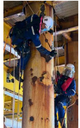
Humidur® FP applied with minimal surface preparation using power tools via abseiling activities on East Belulut Platform in May 2025
