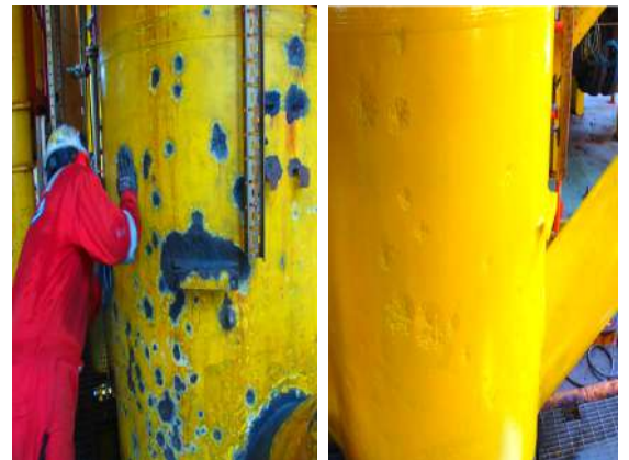
Humidur® FP used for maintenance painting on Bunga Orchid A & E (BO-A, BO-E) Oil Platform, Offshore Malaysia/Vietnam in September 2023. This was done with minimal surface preparation, eliminating need for shutdown of services for repair works.
