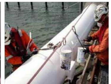
Humidur® FP products used for coating and repair of >100,000m 2 jetty structure and pipes using minimal surface preparation (dry ice blasting) during SPR2 Project at U 7200 in Brunei Darussalam from November 2017 - 2019
