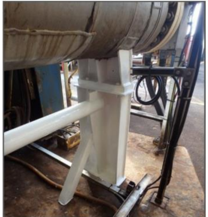
Support of vessel coated with Humidur®
