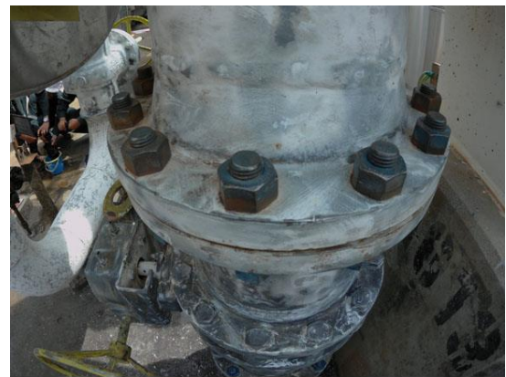
Mechanical preparation to ST2
