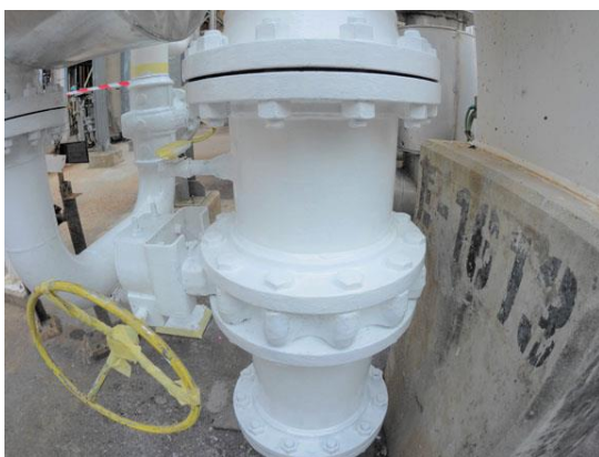
Coating applied during normal surface temperature
