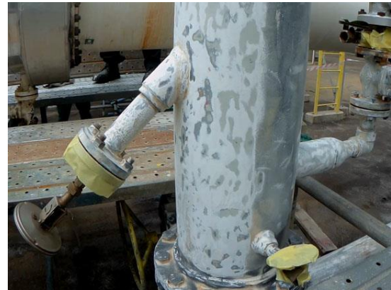
Mechanical preparation to ST2
