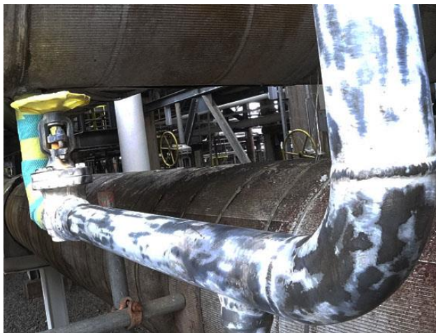
Mechanical preparation to ST2
