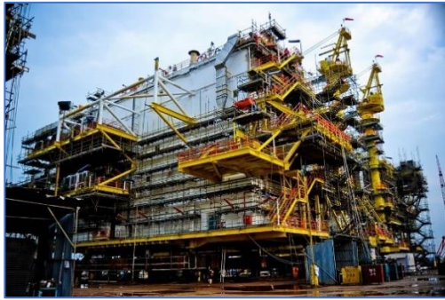
KUMANG CLUSTER Development Project (2008)
