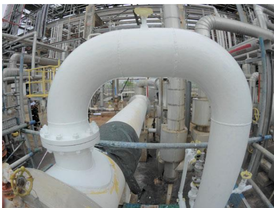
Coating applied during hot surface temperature
