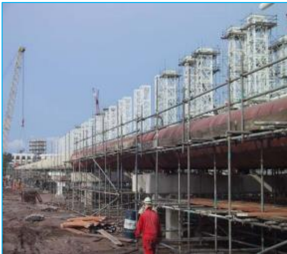
MLNG 3 SLUGCATCHER PROJECT
