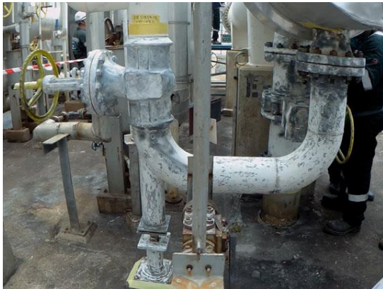
Mechanical preparation to ST2
