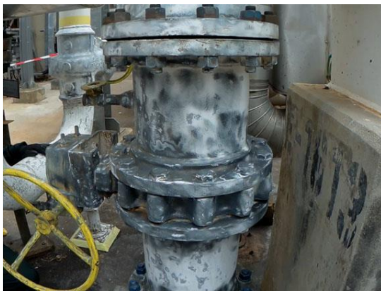
Mechanical preparation to ST2
