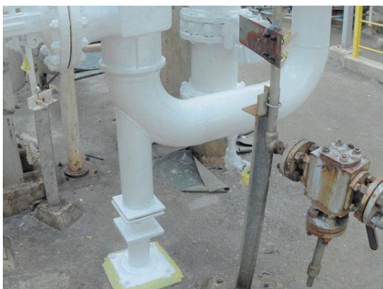
Coating applied during hot surface temperature
