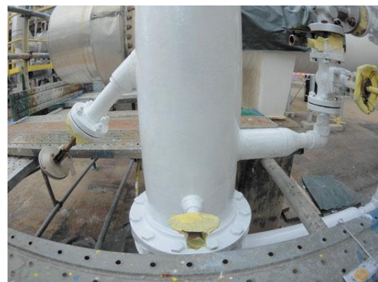
Coating applied during hot surface temperature
