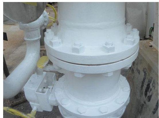
Coating applied during normal surface temperature
