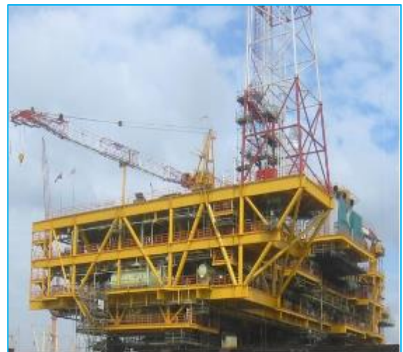
HELANG TOPSIDES PROJECT
