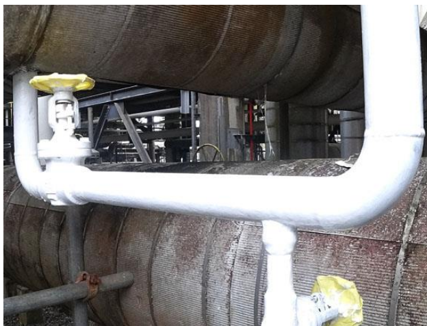
Coating applied during cold surface temperature
