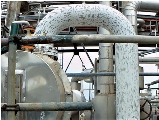
Mechanical preparation to ST2
