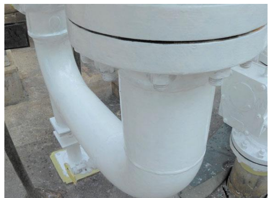
Coating applied during hot surface temperature
