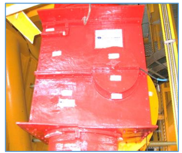
Completed 36" Main SDV, installed and fitted with its PFP castings and wet applied PFP .
