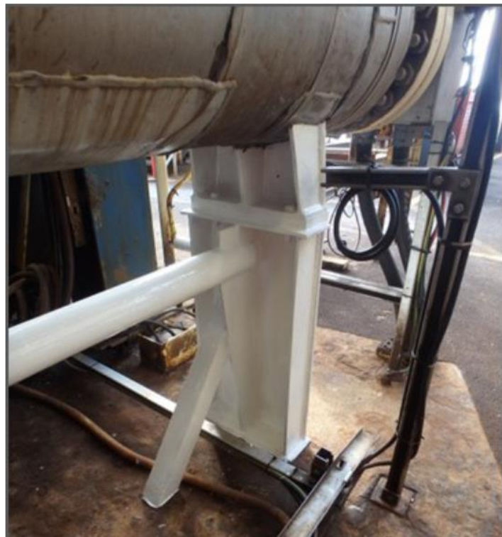
Support of vessel coated with Humidur®
