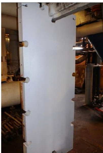
Coating repair with Humidur®
