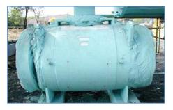
Valve body after wet application. Note, the nameplate and data plate have been left uncovered. They were later covered by removable PFP access panels.
