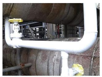
Coating applied during cold surface temperature
