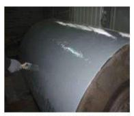
Conveyor belt roller prepared using needle guns and coated with 100MRF Metal Repair Fluid. Bauxite aggregate was incorporated into the wet resin to create an anti slip finish
