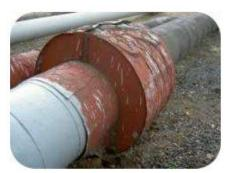
Badly corroded pipe surfaces were hydro-blasted at a European refinery and coated with 2 x coats of ProTXcoat 301 CRSG to give long term protection against CUI
