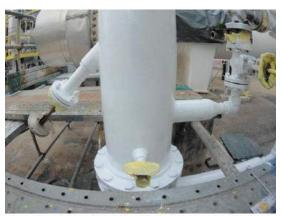
Coating applied during hot surface temperature
