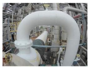
Coating applied during hot surface temperature
