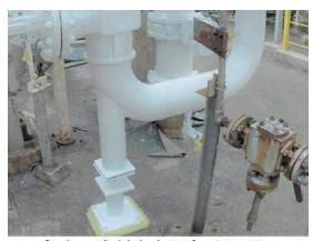
Coating applied during hot surface temperature
